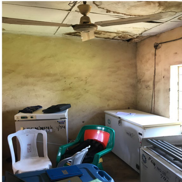
Annex Figure 3: Cold chain equipment in working order but placed under a leaking roof
