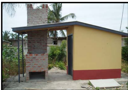
Winneba Hospital Incinerator, May 2007.
